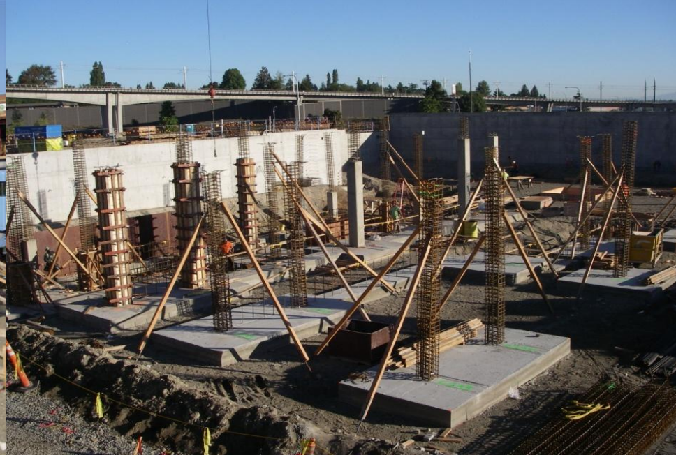
QTA 1 Columns, Footings and Walls
