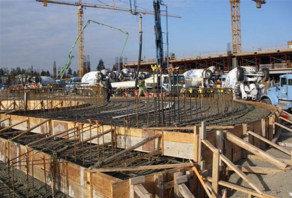
North Helix Placing Concrete
